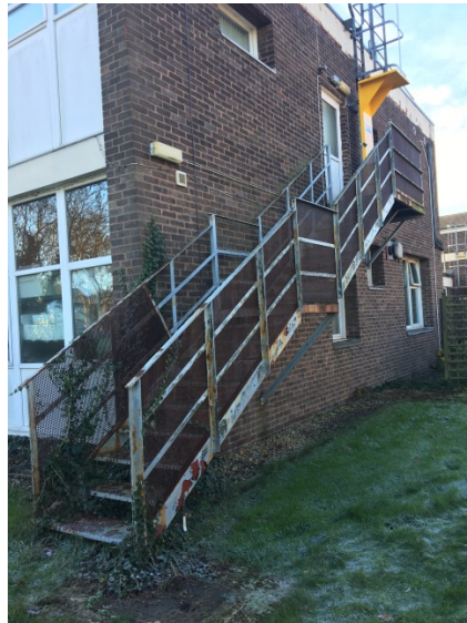
Unprotected External Fire Escape Stair
