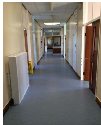
Fire doors requiring replacement
